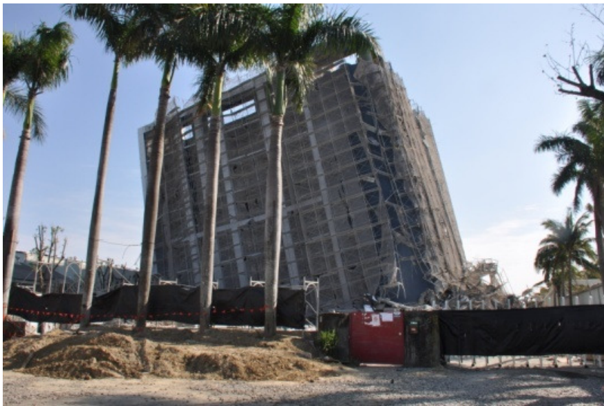
(b) After earthquake
